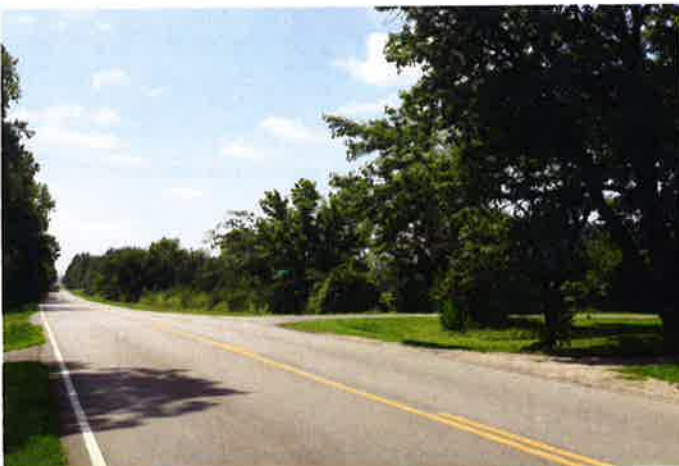
57 TH AVE LOOKING SOUTH
