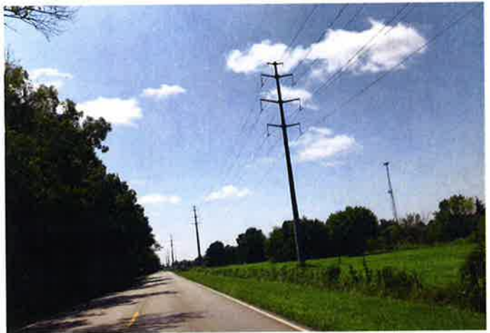
57 TH AVE LOOKING SOUTH
