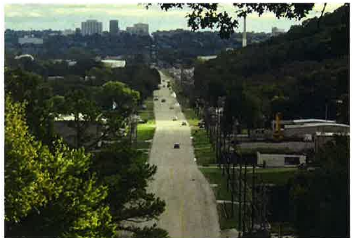
21 ST ST LOOKING EAST
